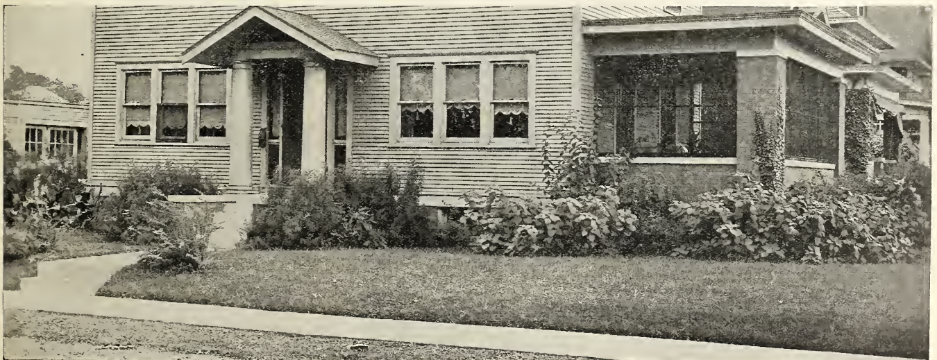
Here is an Effective Planting Binding the House to the Lawn, Softening Angles and Hiding the Low Foundation.
